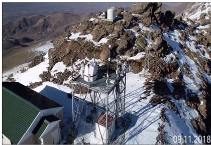
Figure 1 - The tower height is 7 meters and the platform area is 5x5m. The meteorological and astronomical equipment of the DAG-MAM system is located on this tower.
